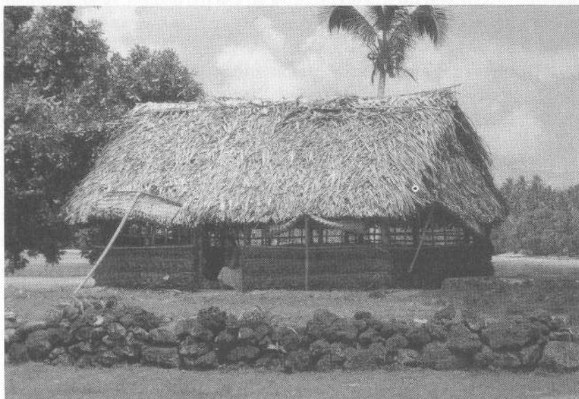
2.2 Thatched Rotuman meeting house showing many elements common to traditional dwellings, though the plaited walls of the latter would be full rather than half height. The rounded ends of the thatched roof, recorded by early nineteenth-century observers, are attributed by Rotumans to Samoan or Tongan influence. Alan Howard, 1960.
